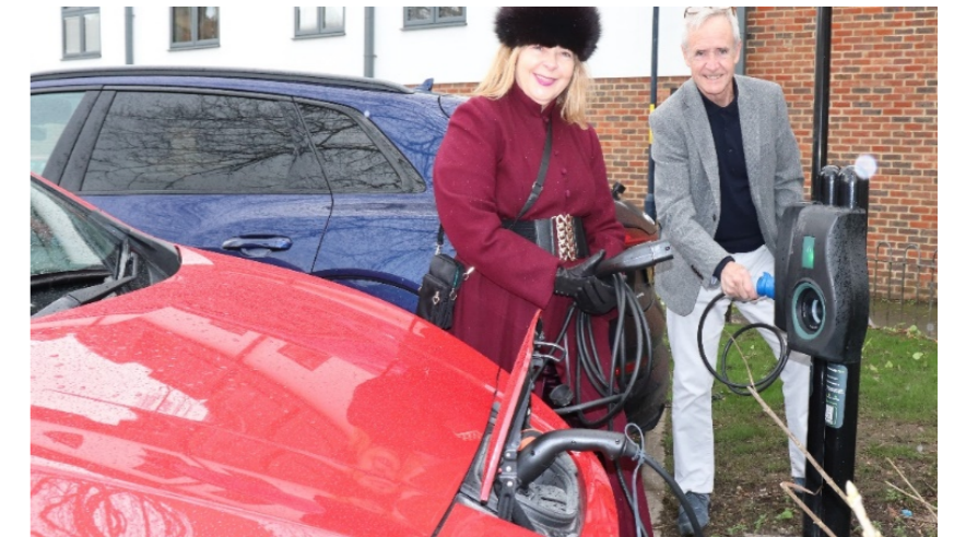
Cllr Susan Carey and Cllr Jim Martin with new EV charging points installed in Hythe.
